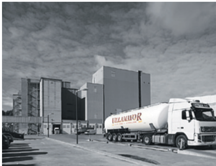
Harineras Villamayor. S.E.
